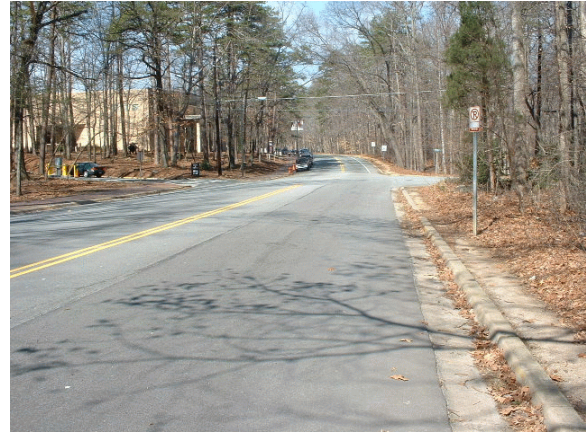
Figure 11. Same road WOL section is clear.
