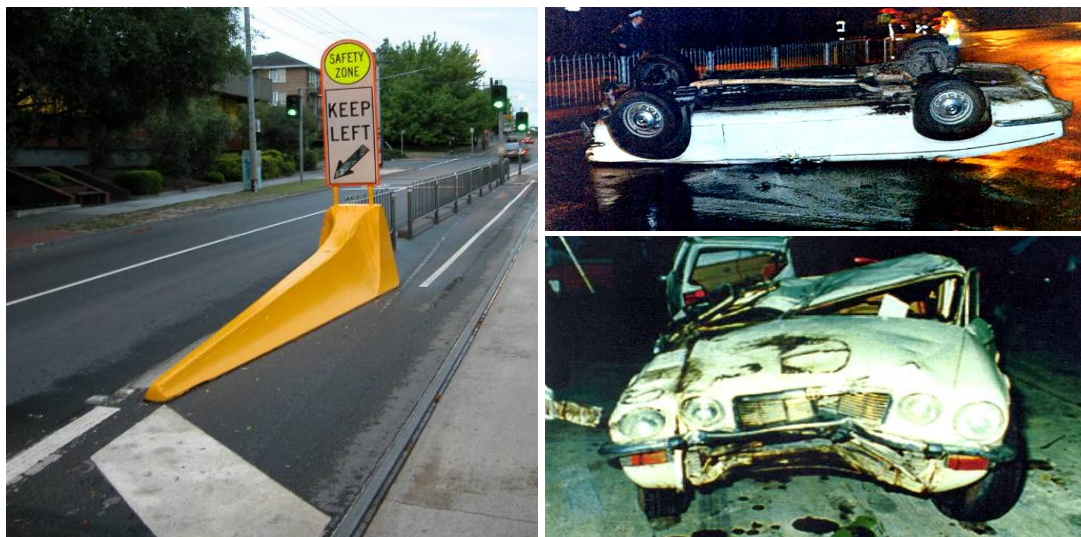
Figure 4 - Tram ramp protects pedestrians but results in vehicle Flip-overs.
